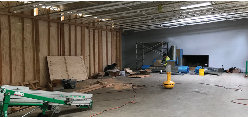
Demo time in the main hall at the Community Center. Flooring, ceiling tiles, and front facade have been removed to prepare for upgrades. Photo by Sylvia Hacaj.
