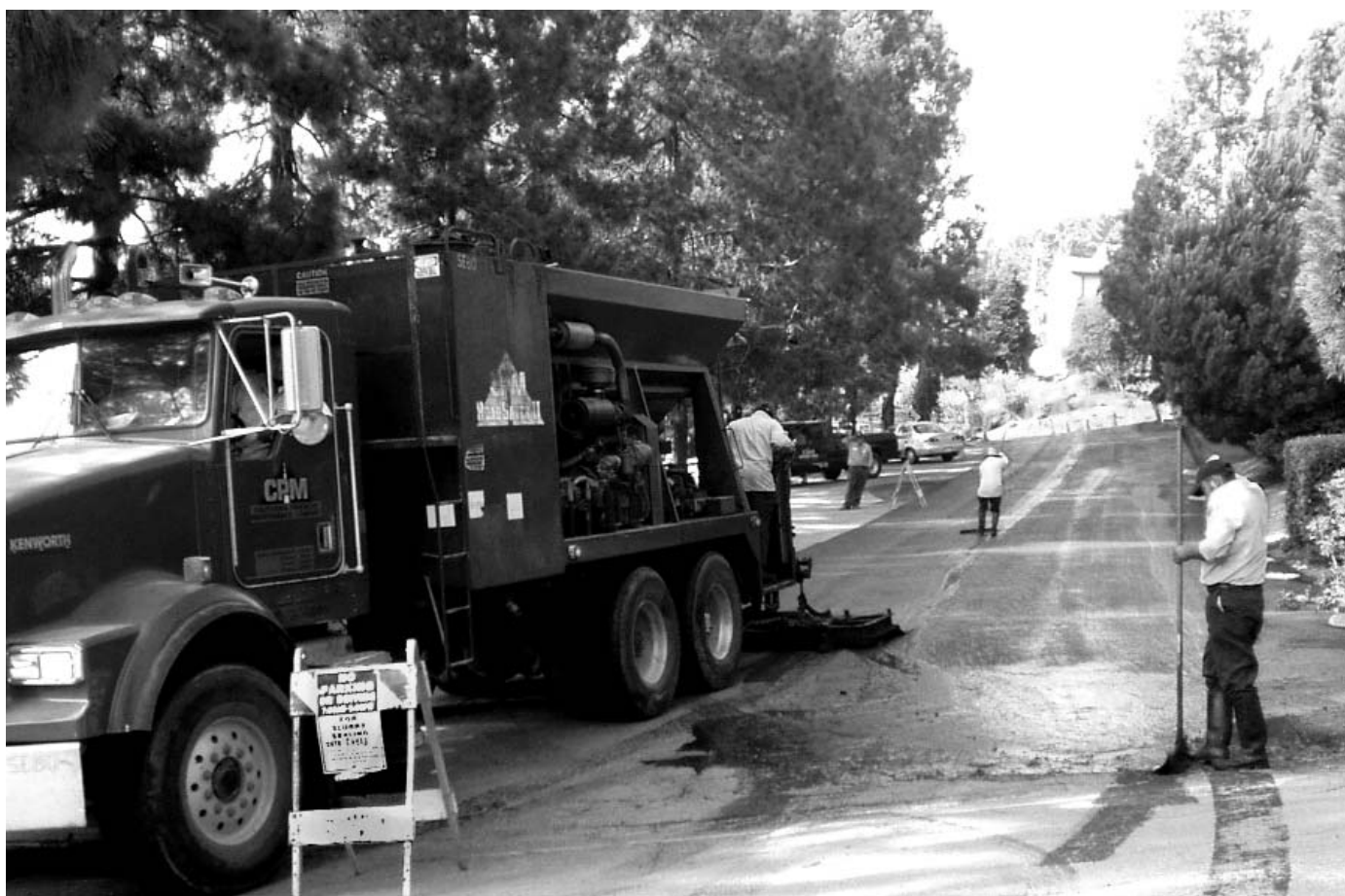
PAVING THE WAY: A work crew from CPM lays down slurry on the parking lot across from the Arlington Community Church.
