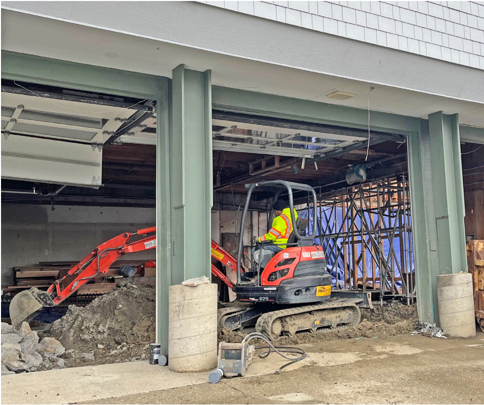
The interior of the Public Safety Building has been torn down to its studs, concrete floor removed, and asbestos abatement completed. The building must be in move-in state by September 1, 2024. Photo by Byron Kawaichi.
